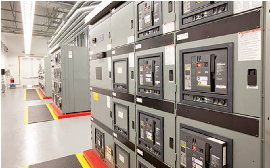
University of Massachusetts Medical Center data information facility, Shrewsbury MA
